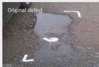
The images on the left show the complete patch repair applied to a defect. Over a 2½ year period, this patch repair has not required any follow-up maintenance – as shown in the bottom image.
