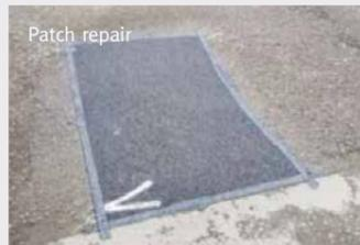
With the particular brand of cold lay material that it uses, Milton Keynes Council can complete permanent planned and emergency repairs on estate roads on potholes and areas up to 2m².
