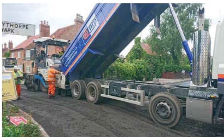
Figure 3. Ultifoam being laid
