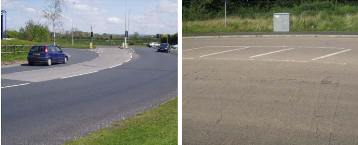
Plates A3.4 & A3.5 High Friction Surfacing - Used at the approach to junctions, crossings and on bends
