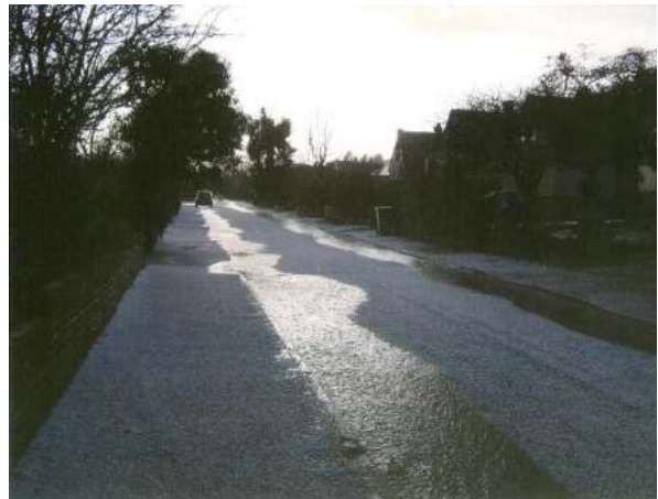
Plates 45a/b: Urban flooding – inadequate capacity and inadequate edge collection
