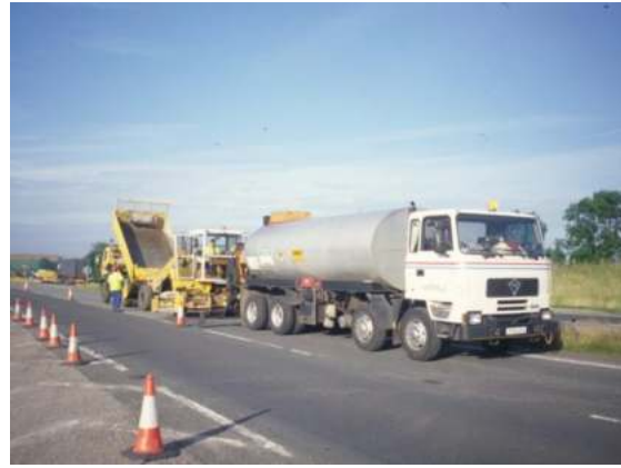
Plate A4.4 Surface Dressing – Sprayer with chipper behind
