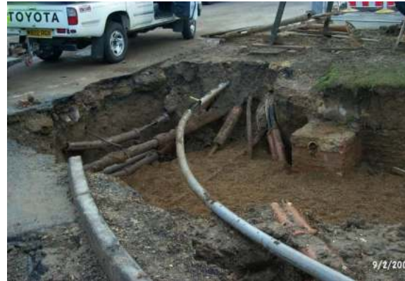
Plate 38: Mineworking collapse
