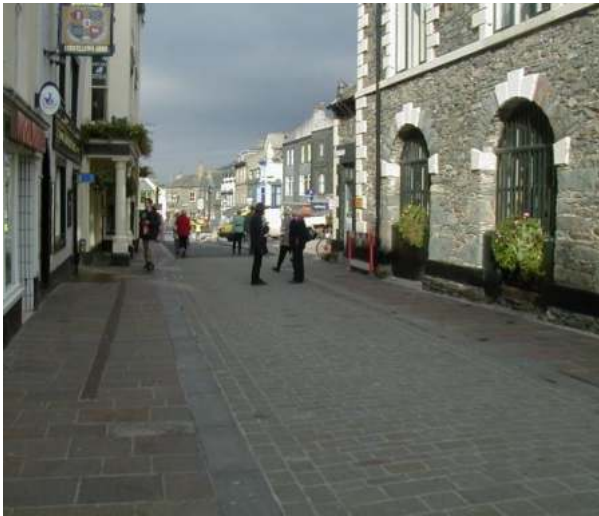
Plate A7.1 Modular pavement in Keswick Town Centre
