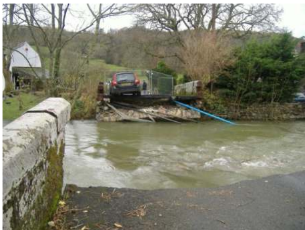
Plate 3.1 Lorton Bridge, Cockermouth, Cumbria
