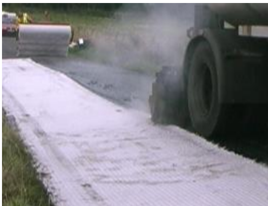
Plate 58: Steel mesh reinforcement [49]
