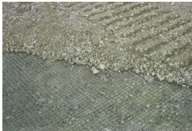
Plate 61: Polypropylene grid reinforcement [51]
