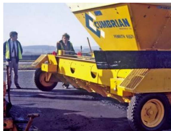
Chipper to uniformly spread the “pre-coated chippings”
