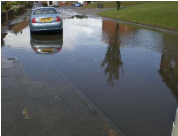
Plates 45a/b: Urban flooding – inadequate capacity and inadequate edge collection
