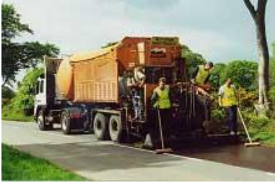
Plates A4.1 & A4.2 Slurry surfacing
