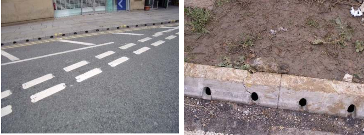
Plates 57: Linear kerb drainage channels
