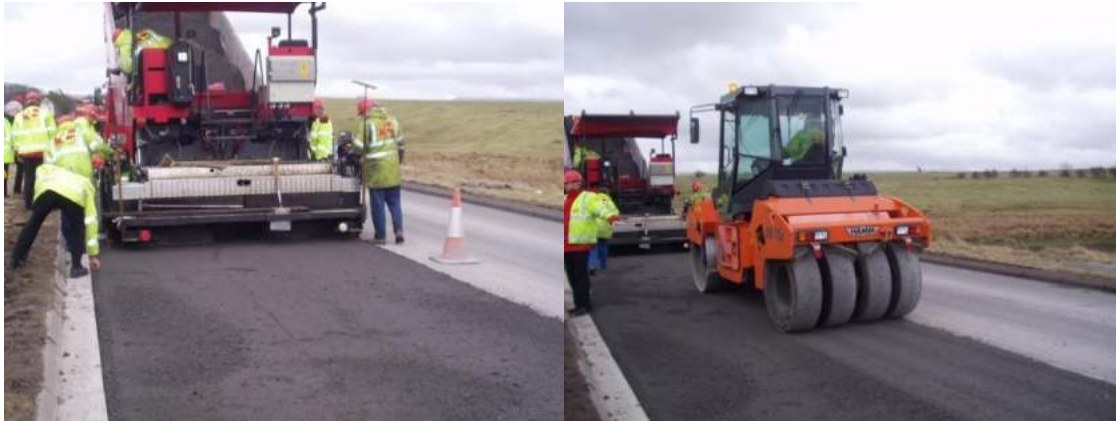
Plates A3.8 & A3.9 Recycled material used as binder course
