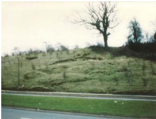
Plates 41: Examples of slope instability
