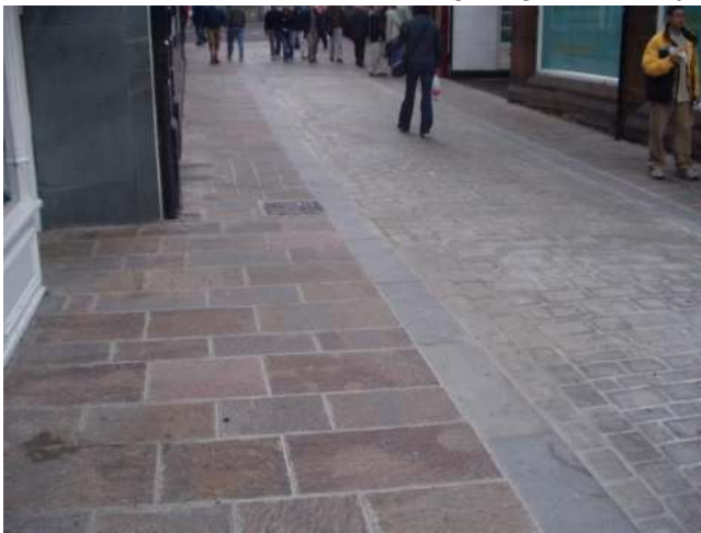
Plate A9.1 Modular footway in Keswick Town Centre
