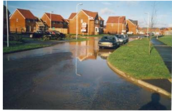
Plate 47: Inadequate drainage due to inadequate road sweeping
