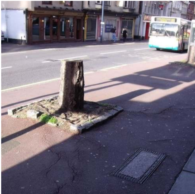
Plate 62: Removing footway distress trees
