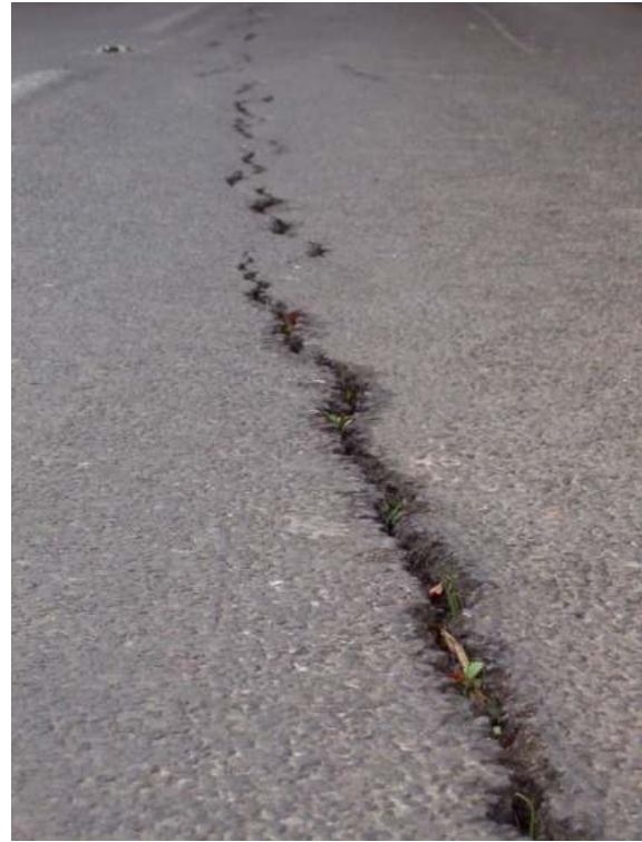
Plates 16: Carriageway distress due to peat desiccation
