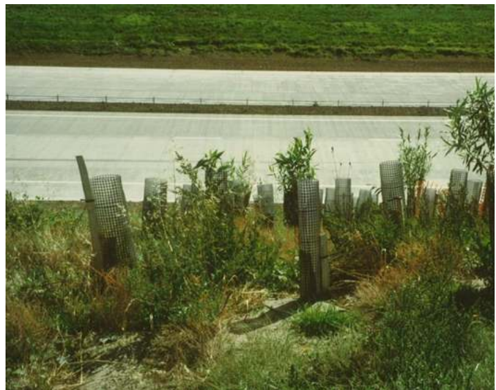
Plate 21: Live willows to improve slope stability
