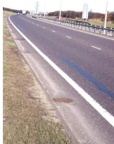
Plates 6 and 7: Longitudinal carriageway cracking on a clay soil
