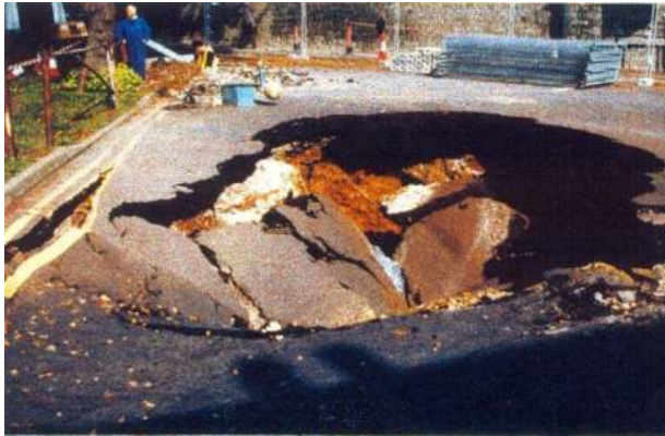
Plate 37: Collapse settlement
