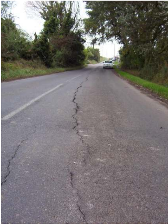
Plates 16: Carriageway distress due to peat desiccation
