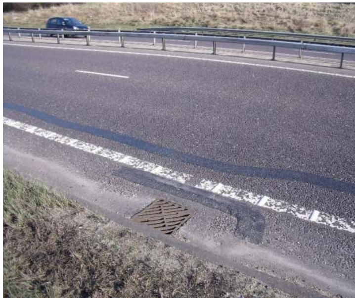
Plates 6 and 7: Longitudinal carriageway cracking on a clay soil
