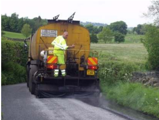
Plate A4.3 Surface Dressing – Sprayer carrying out “quartering” operation
