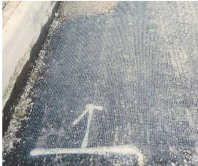
Plate 59: Glass fibre reinforced mesh [50]
