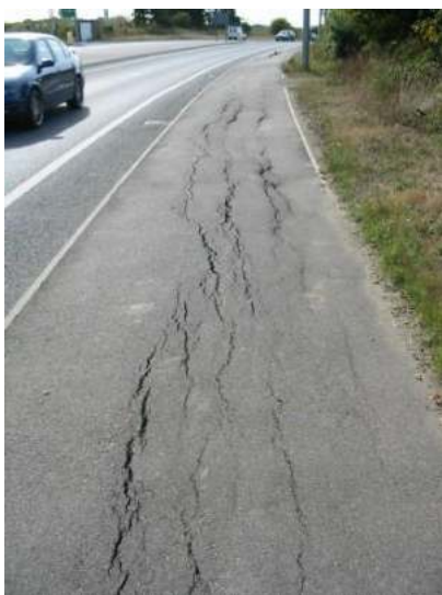
Plates 3: Footway desiccation cracks
