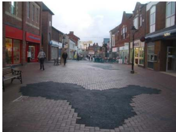
Plate A7.2 Limited repair options once modular pavements fail
